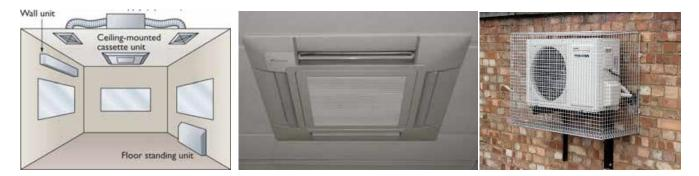
It should be noted that locations with Air Source, Ground Source Heat Pumps will have visually similar external equipment and the Service Records should be consulted to determine the type installed.
